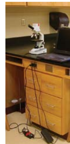
Not enough outlets— a real safety hazard
