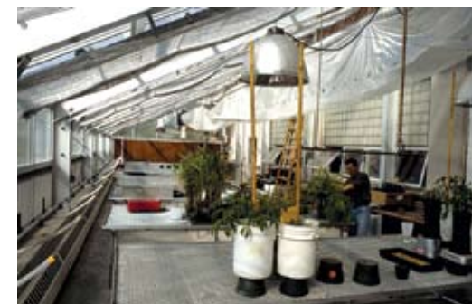
Well-ventilated greenhouse with both a fan system and operable wall panels
