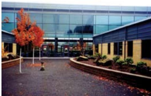
Courtyard with permeable paving
